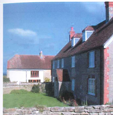
The original stone Coach Road Farm was extended on the right side in the 19th century; here the stone facing has brick detailing around the windows, along the bottom of the wall, and edging on the corner. In the centre of the facade is a gabled wooden porch with a tiled roof. In 2005 a further extension was built onto the rear to form a T-shaped building. Coach Road Barn can be seen in the background.
